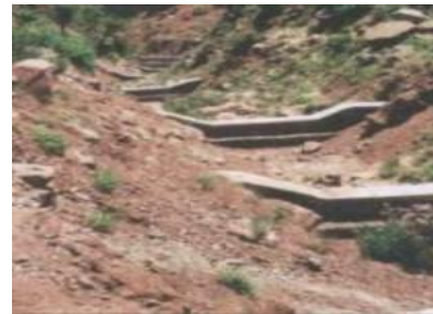
Check dam – cemented stones, for the protection of the ravine in the Taza basin (Source: Berhailli)
