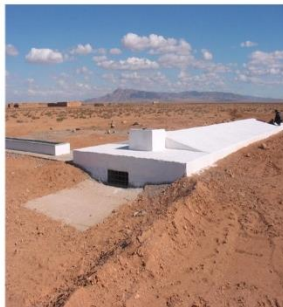
Concrete tanks (Matfias) open/closed, buried/semi-buried (M.Kharmouch)
