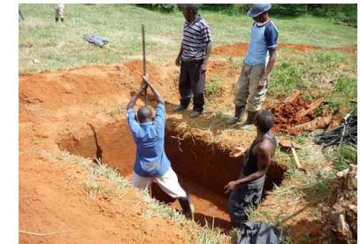
Constructing a tube recharge system (Connect International)
