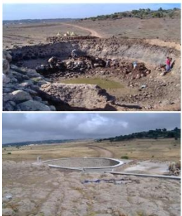
Concrete tanks (Matfias) open/closed, buried/semi-buried (M.Kharmouch)
