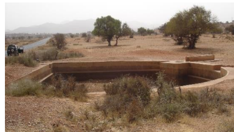
Surface water reservoir (Matfia) fed by a road, Morocco (Source: M. Sabir)
